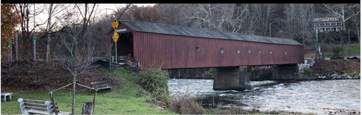
Historic Cornwall Covered Bridge
