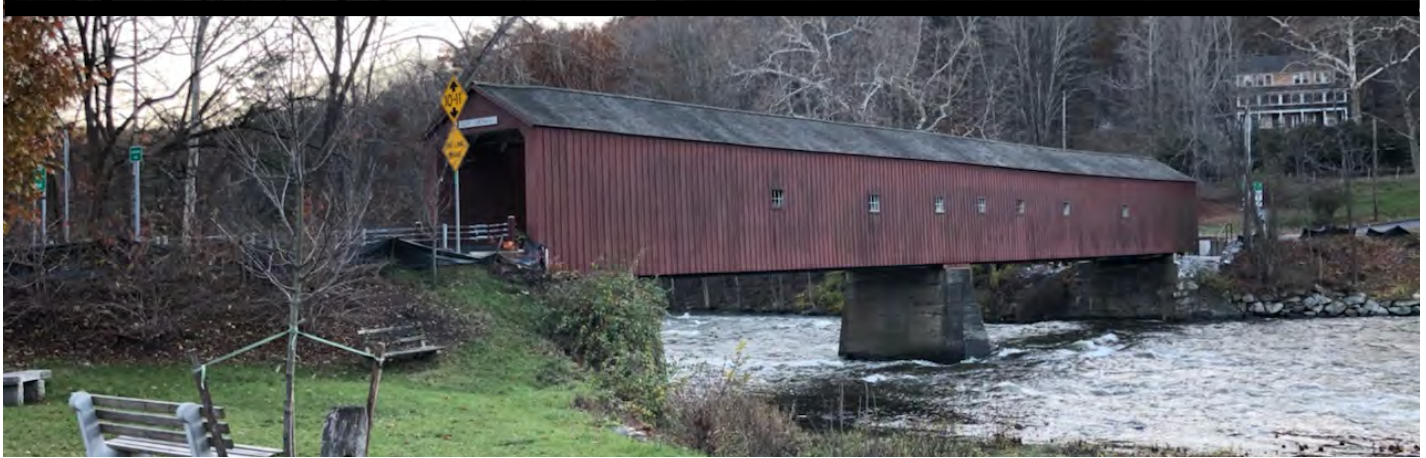
Historic Cornwall Covered Bridge
