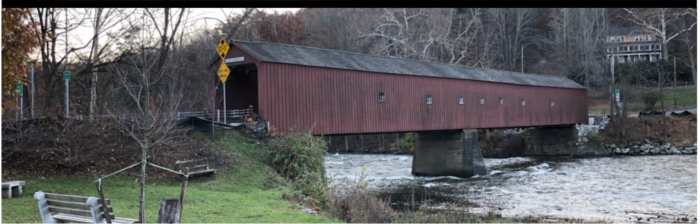
Historic Cornwall Covered Bridge
